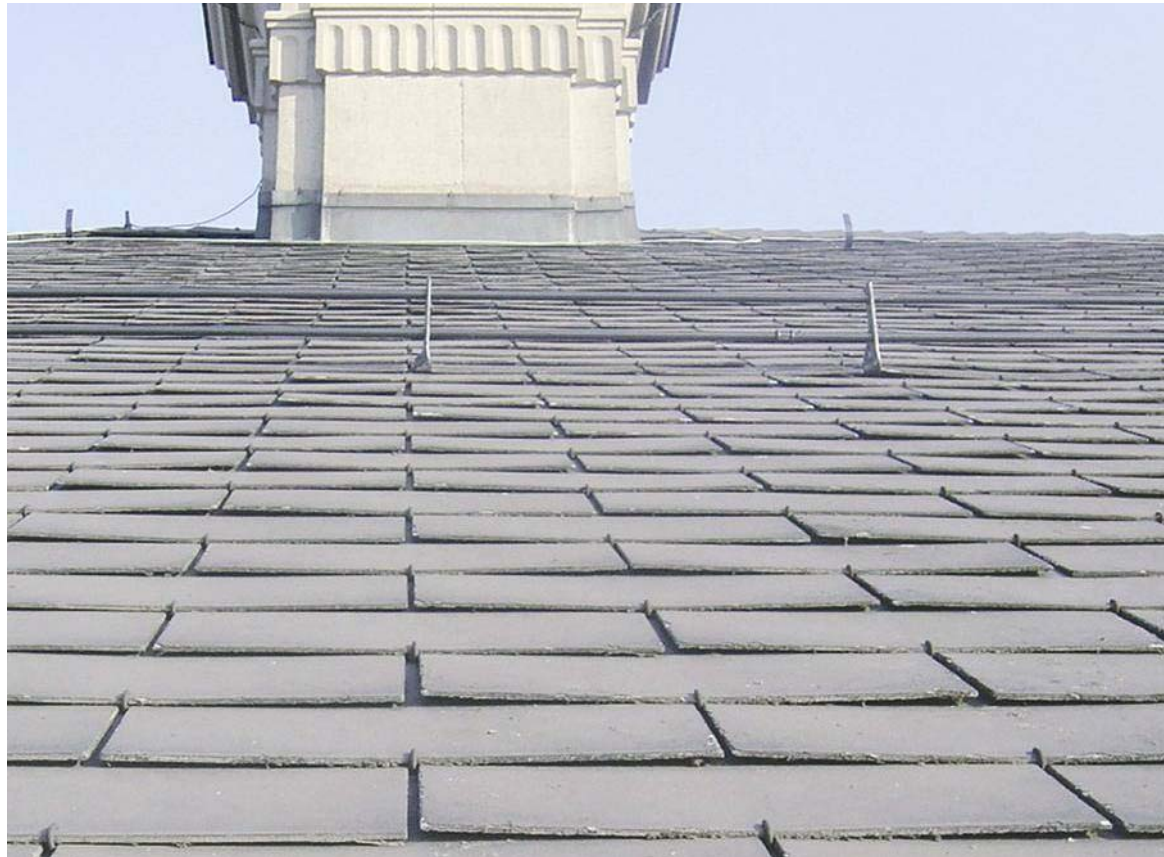
Scandole in cemento-amianto
